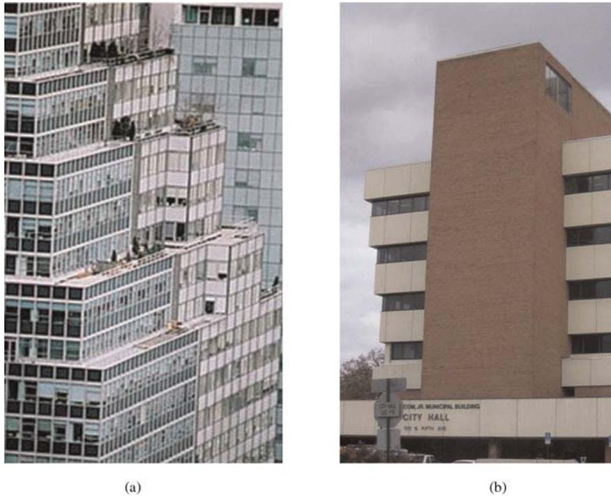
**Fig. 1.** A comparison of the “stacked” building construction: (a) a traditional form, which is commercial building from Jeff Klamer Design, and (b) a “flipped” form, which is the Ann Arbor, Michigan, City Hall Building. [A color version of this figure can be viewed online at [journals.cambridge.org/aie](http://journals.cambridge.org/aie)]
